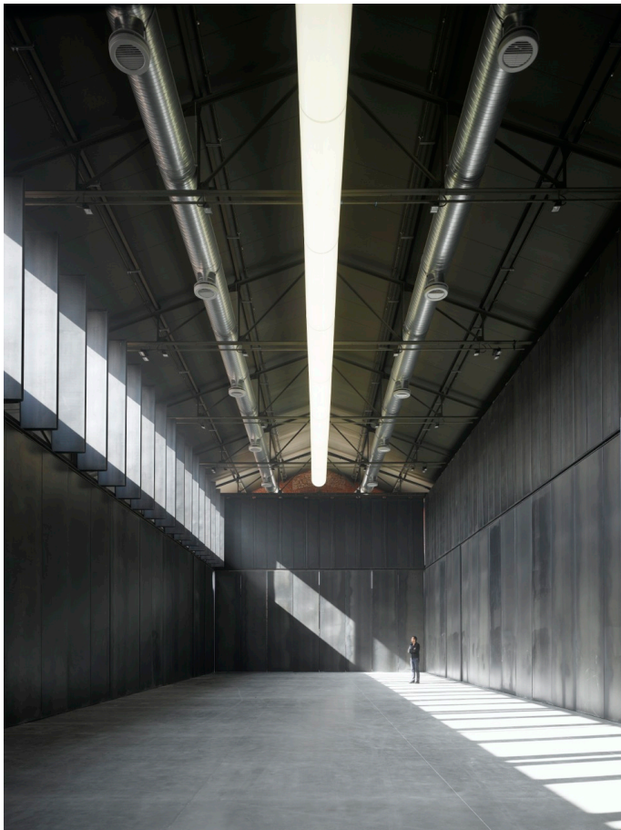
Hangar 16 Matadero-Madrid (Slaughter House-Madrid) by Iñiqui Carnicero Arquitectos © Photo by Roland Halbe.
